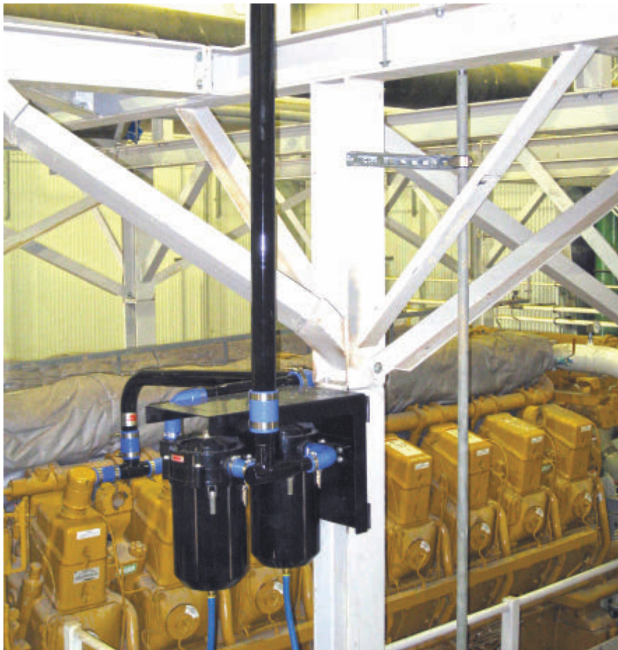
Two Racor CCV12000 crankcase filters are shown, attached to a Caterpillar 3616.
